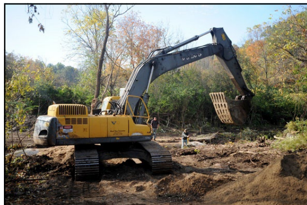
A work crew installs a culvert as part of the Malletts Creek restoration project. The culvert is being put in to help stream flows and reduce flooding.
